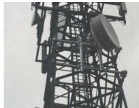
Licenced microwave is the ideal technology for long primary backbone links. Distances in the tens of kilometres are possible. This is the technology upon which 90% of the cellular networks are based.
